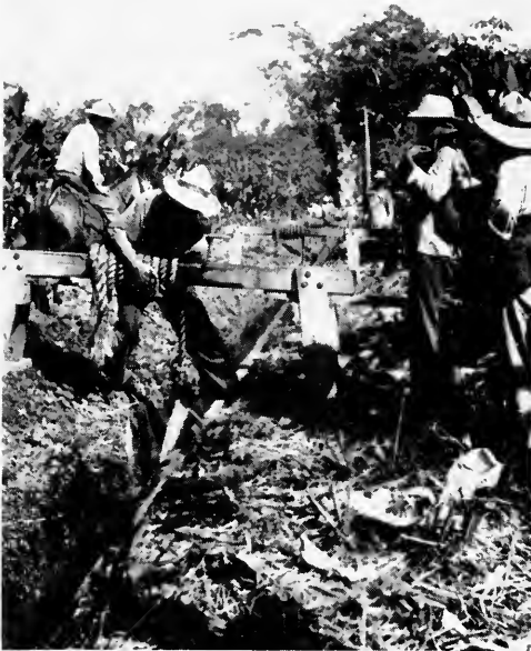
LOWERING PIPE INTO DITCH
